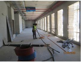
Celling Mechanical and Electrical first fix ongoing in Block 1 August 2020.
