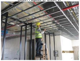
False celling works ongoing on the ground floor of Block 1 during November 2020.
