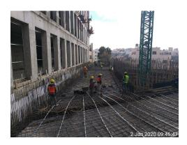
Roof slab reinforcement and shuttering works in Block 4.
